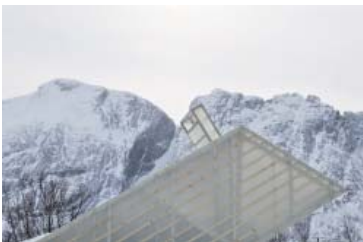
Jektvik Toilett, kiosk and ferry area, Helgelandskysten Tourist Road. 2010
